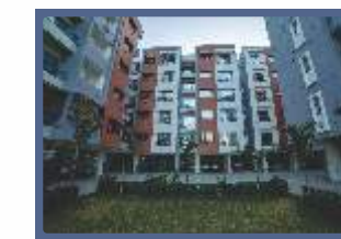
SAMANVAY SPARSH RESIDENTIAL APARTMENTS @ VADSAR KALALI MAIN ROAD
